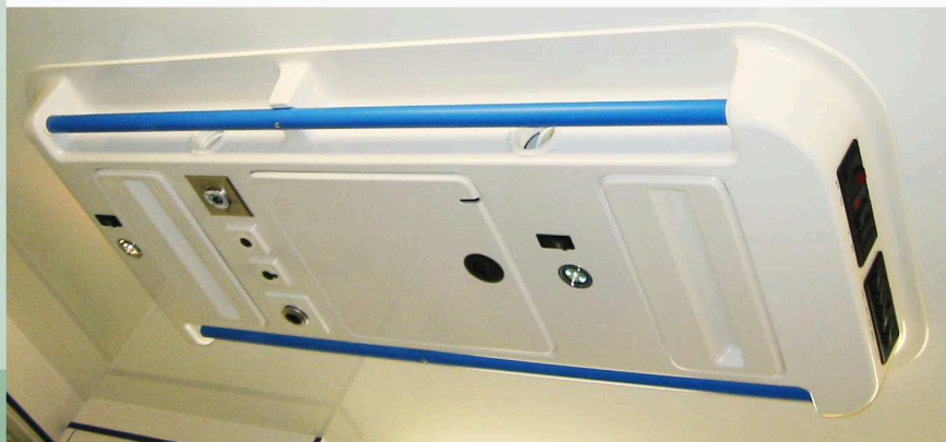
Dome mounted central-supplying-center with integrated handrails, various compartments for e.g. oxygen equipment, infusion bottles and ECG-supply. At the front is place to mount operating switches for the patients table and other electrical devices (e.g. lightning)
